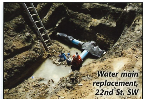
Water main replacement on 22nd St. SW
